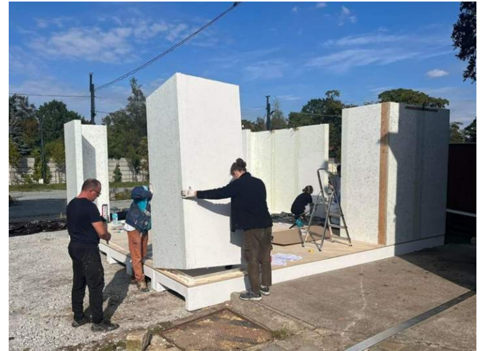
Construction at site
