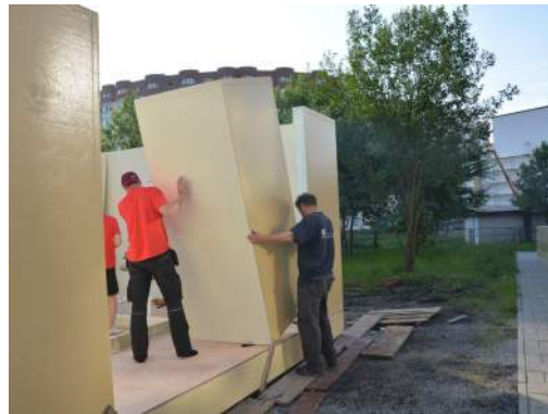
Construction at site
