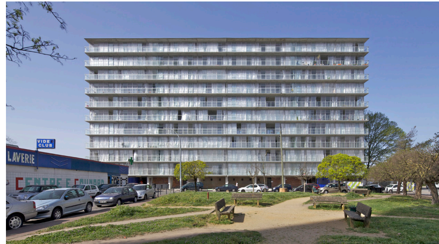
New facade. Soucre: Lacanton Vassal
