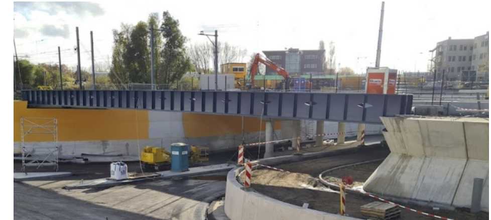
Here the circular concrete mixture produced by Rutte Group with the help of SmartCrusher technology is used in a reinforced concrete component that separates the road from the cycle path. Source: slimbreker.nl, 2022
