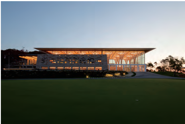
Timber Structure: Haesley Nine Bridges Golf Clubhouse Yeosu, Korea (2010)
