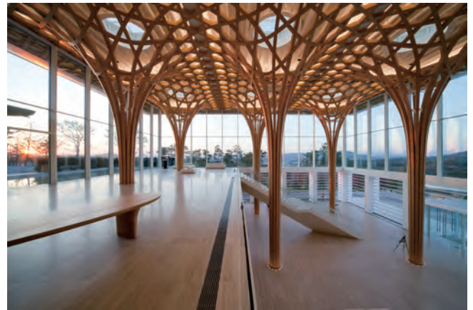
Haesley Nine Bridges Golf Clubhouse – interior
