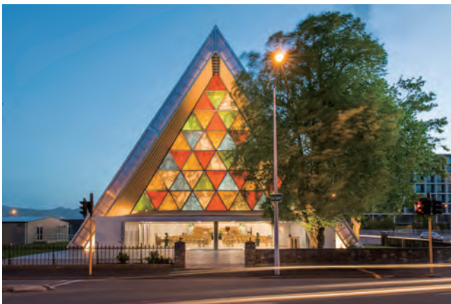
Cardboard Cathedral for 2011 Christchurch Earthquake (2013)
