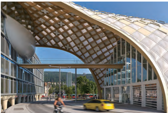
Timber Structure: Swatch Omega Biel/Bienne, Switzerland (2019)
