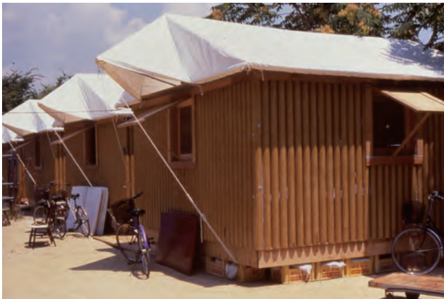
Paper Log House Kobe for Hanshin Awaji Earthquake, Hyogo, Japan (1995)
